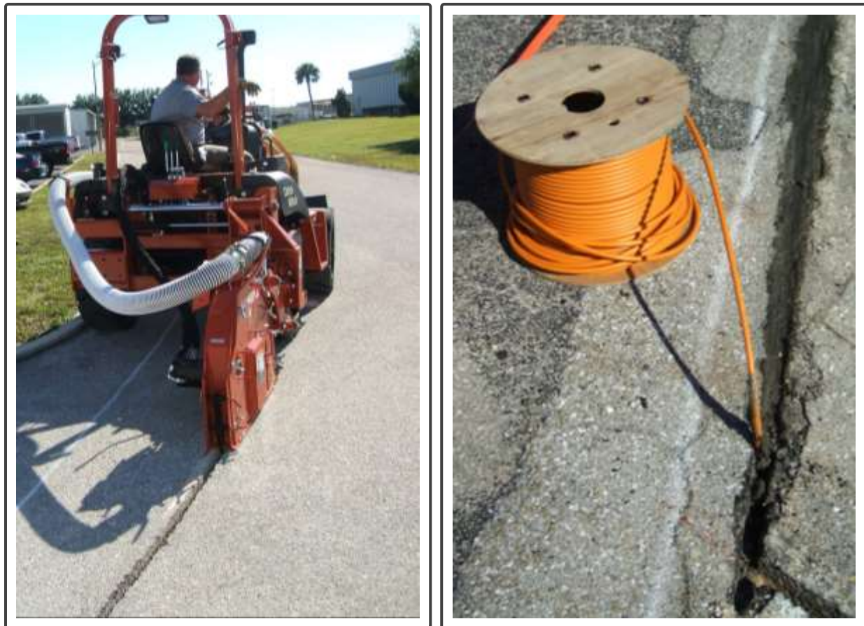
Figure 2-26. Microtrenching
