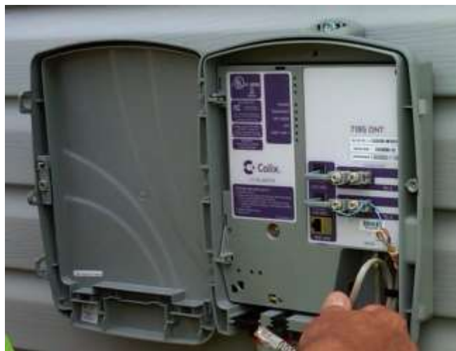
Figure 2-22. Small Fiber Termination Box with Exterior Ethernet Switch
